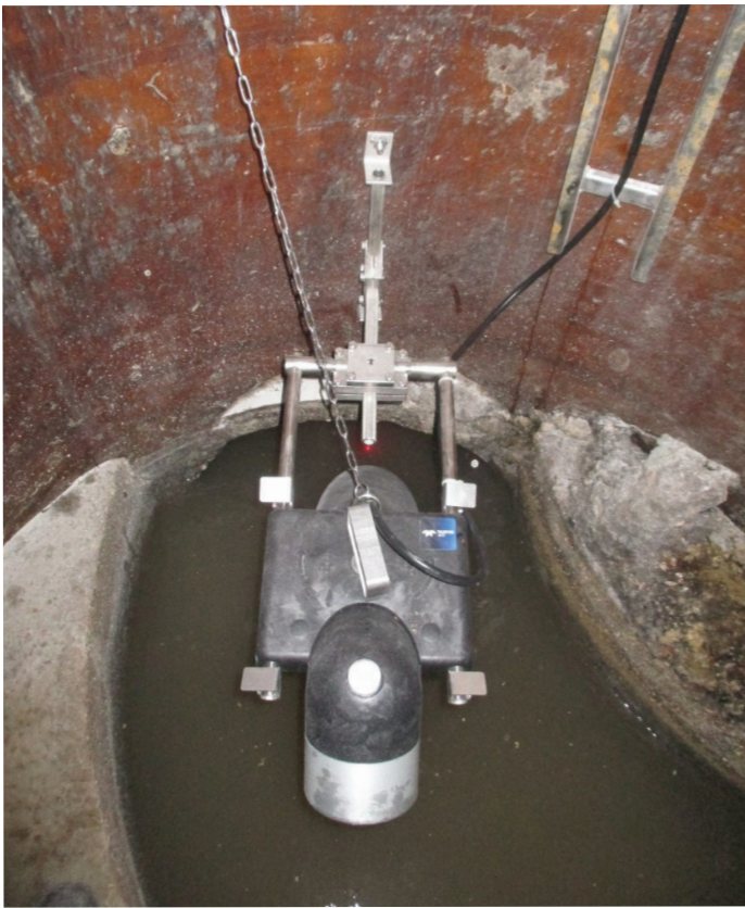
Figure 2: Sensor installation in the manhole.
